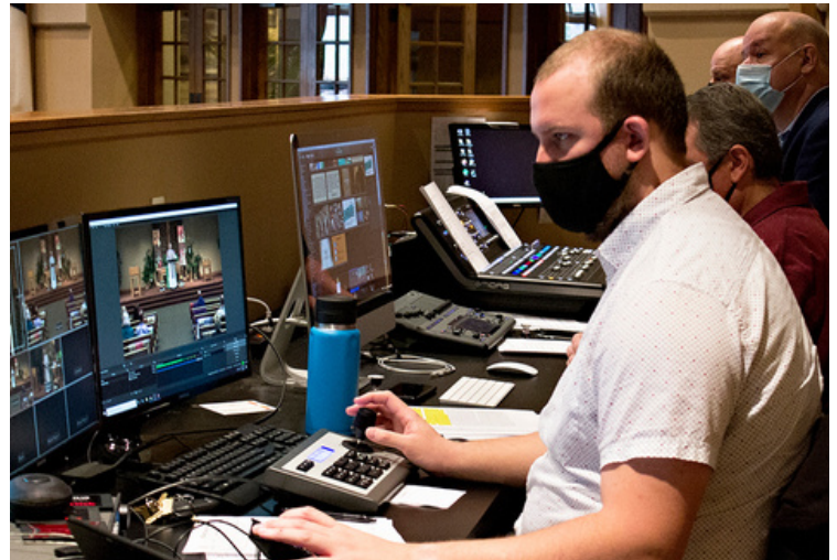
Livestream equipment was installed in both worship spaces in October in order to improve online ministry and service experiences.
